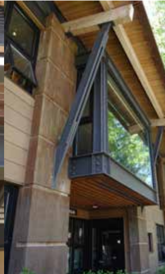
Framing connections
